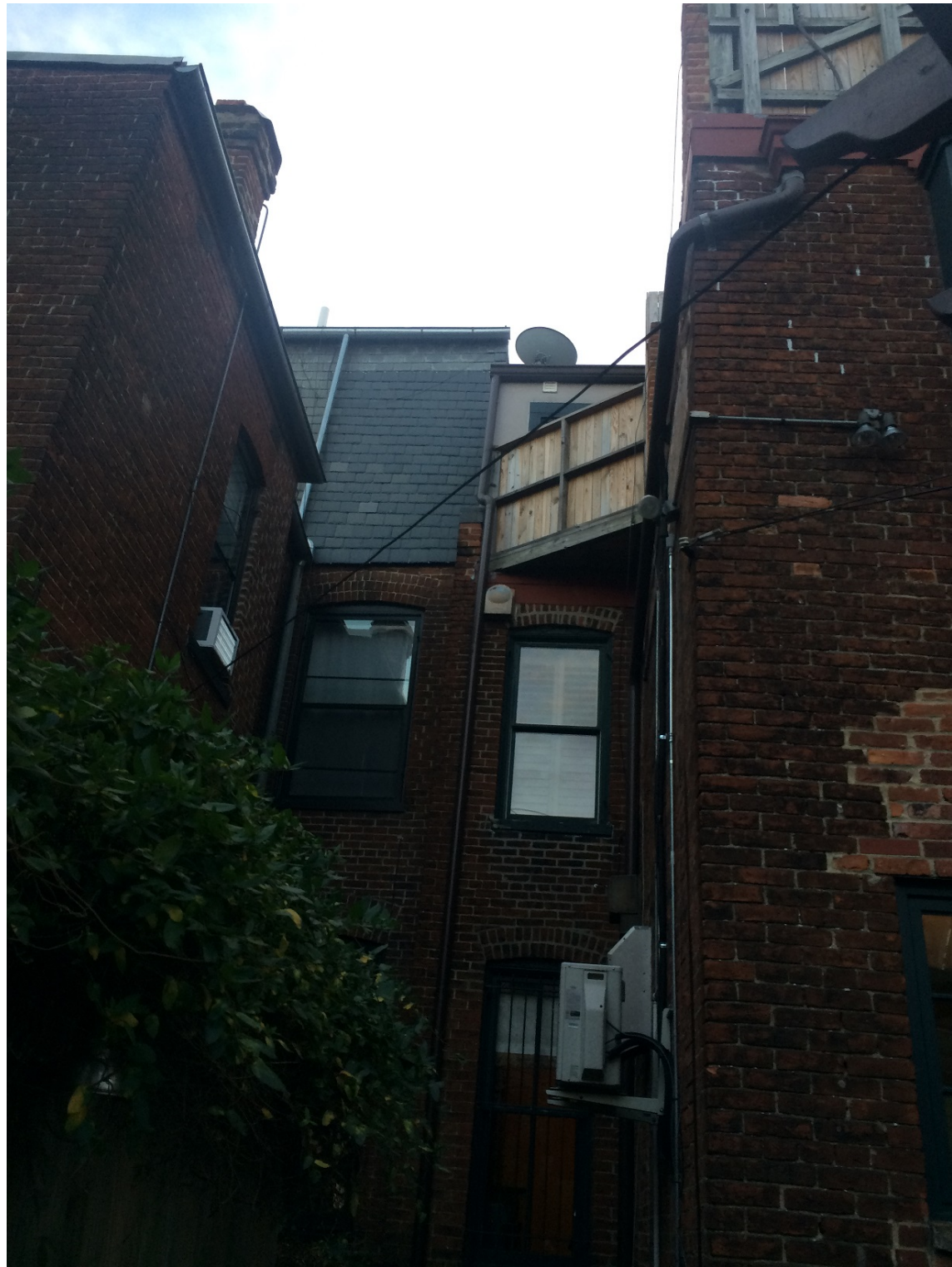
VIEW OF EXISTING DOGLEG @ 1016 MASSACHUSETTS AVENUE SE
