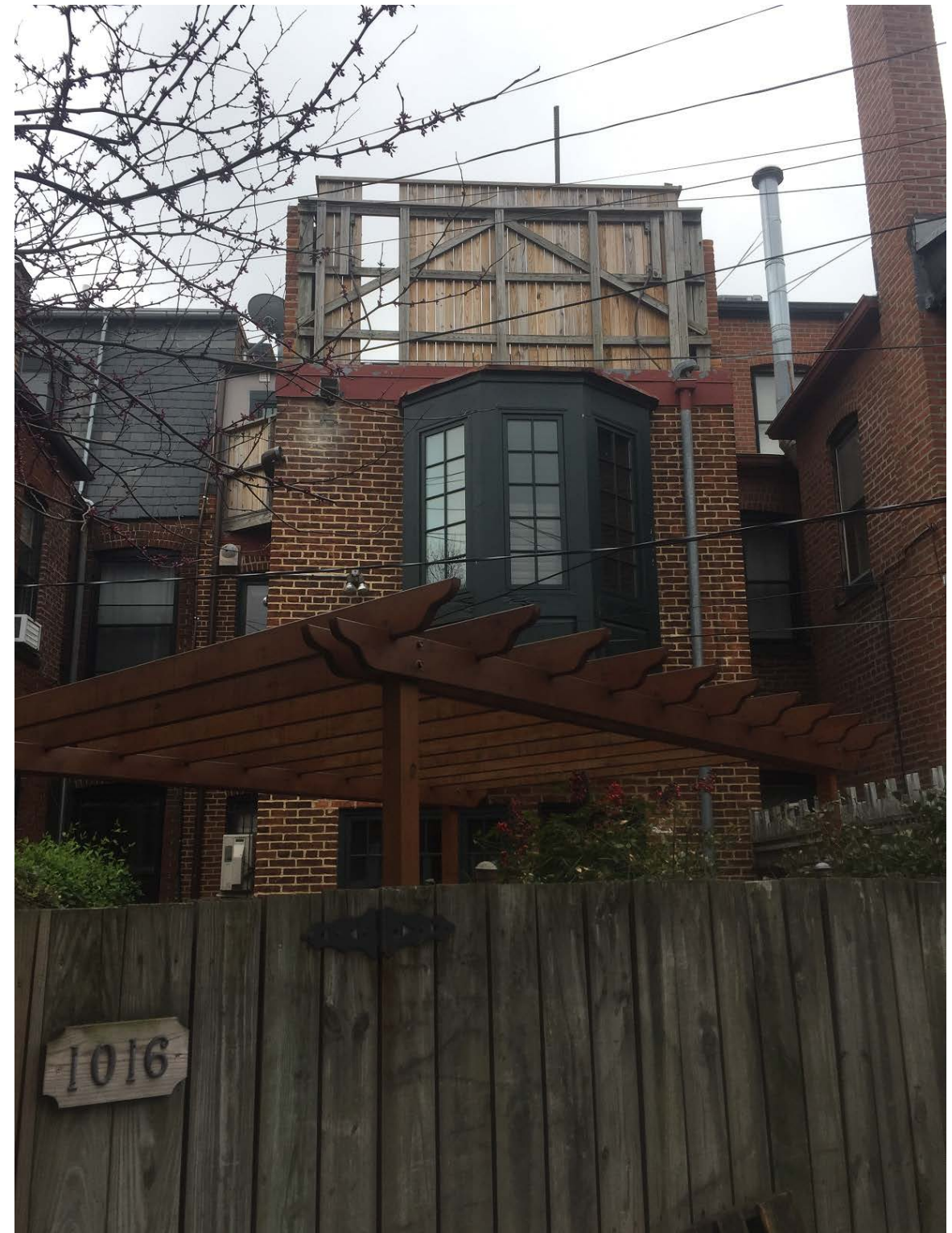
VIEW FROM ALLEY OF EXISTING REAR FACADE
