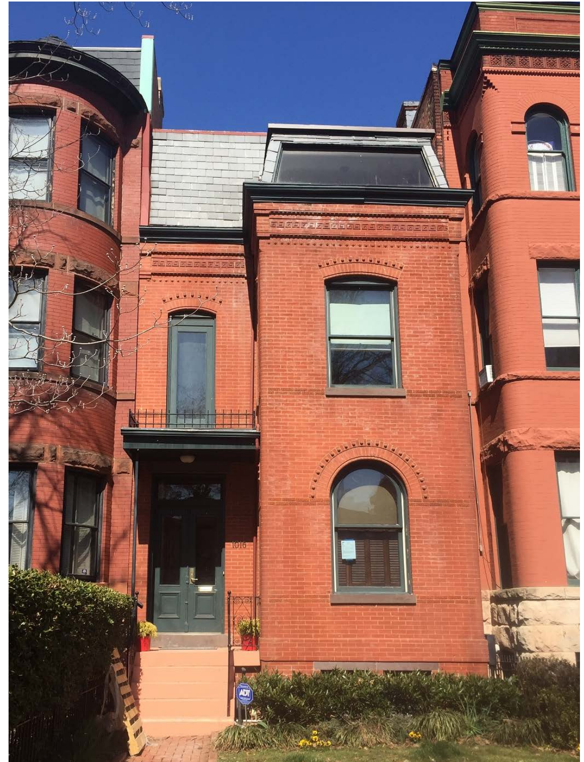
EXISTING FRONT FAÇADE
